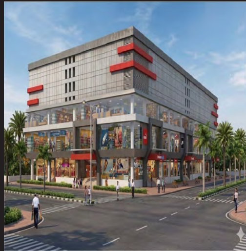
Shalimar Miracle Goregaon
